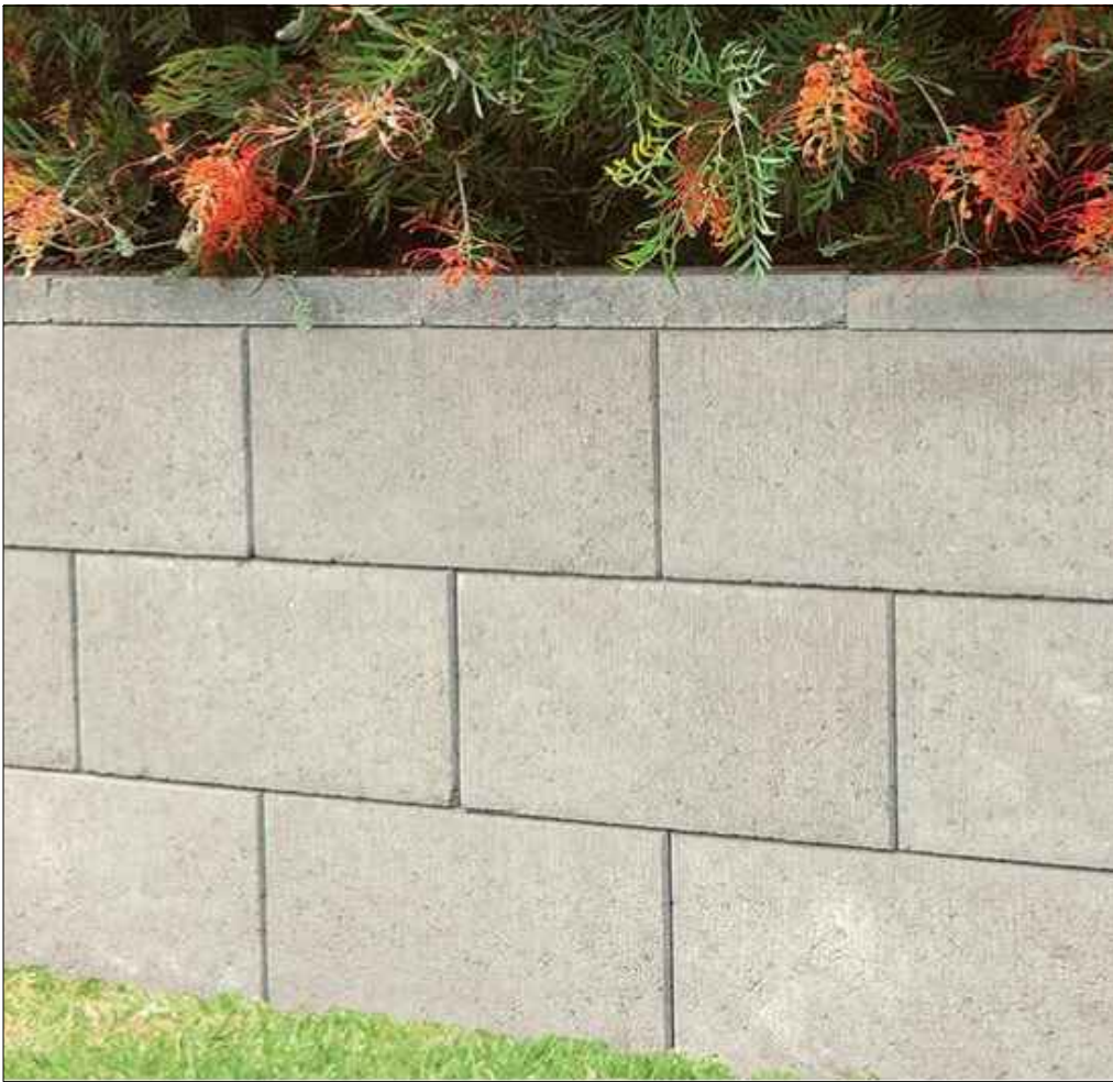
WAL-1 CONCRETE BLOCK RETAINING WALL ADBRI MASONRY 'VERSALOC' CONCRETE BLOCK 400x190x200 NATURAL FINISH OR SIMILAR
